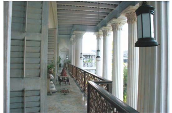
A view of the first floor verandah
